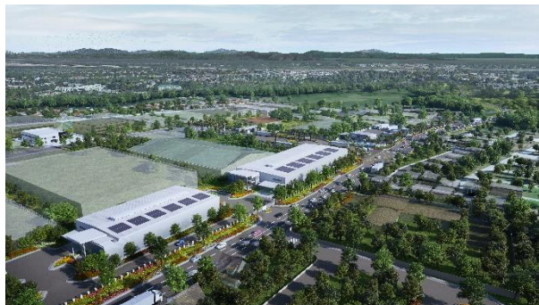
Photo caption: RBF Industrial Strip in FIP NCC
